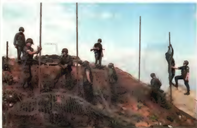
Marines erecting a fence at their Beirut compound this month to deflect bomb fragments
